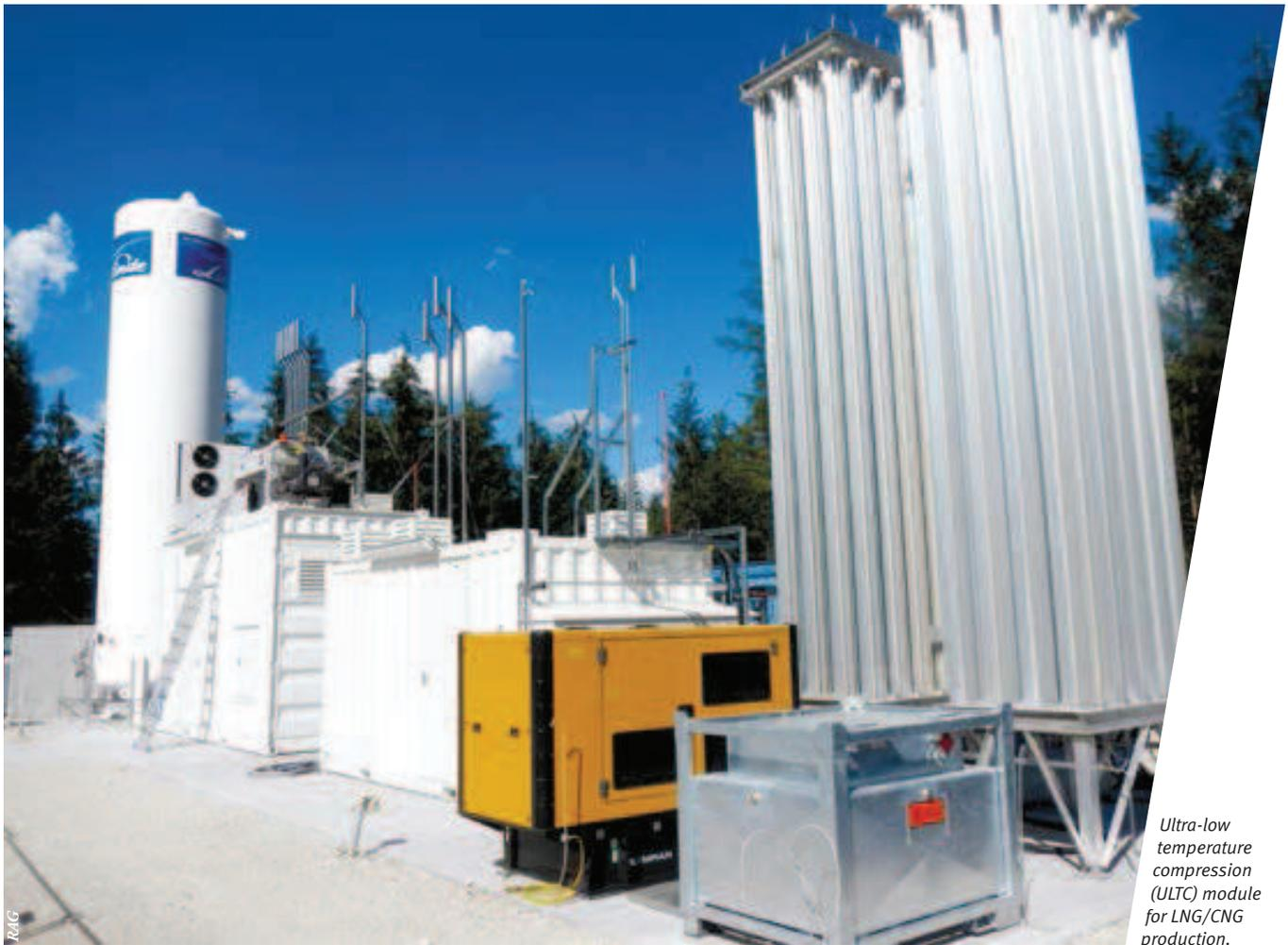
*Ultra-low temperature compression (ULTC) module for LNG/CNG production.*
